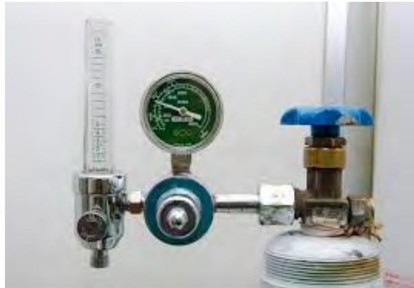
**FIGURA 3.** MANÓMETRO O MANORREDUCTOR.
